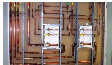
Typical commercial medical gas installation rough-in.
